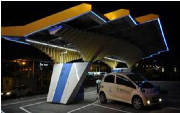
Figure 7-8: SRTPV powered charging station
