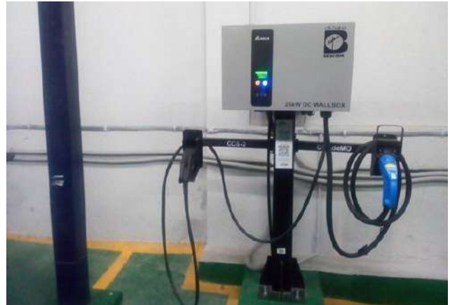
Figure 1-1: Fast DC - CCS/CHAdeMO charger
